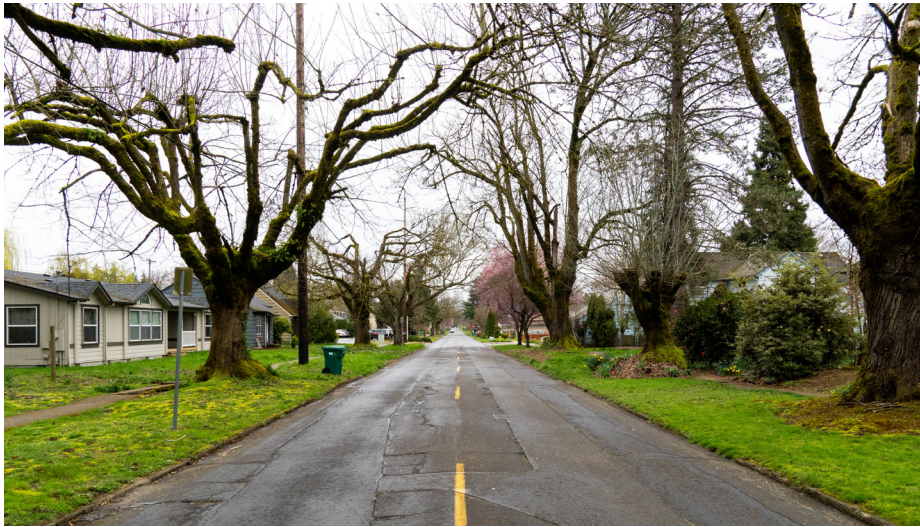
River Street is “the worst road in Newberg,” according to city officials. They presented design options to completely rebuild the street on March 9. (Branden Andersen / Newsberg)
